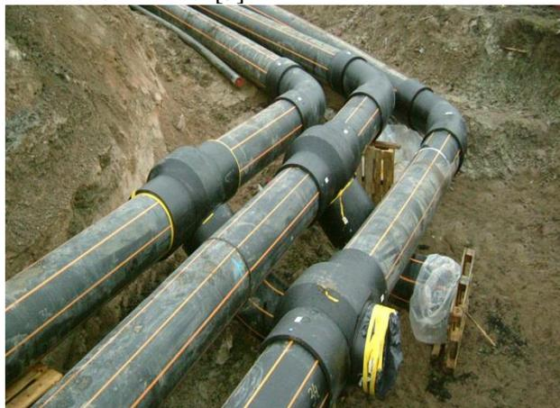
**Figure 1.** Assemblies of polyethylene fittings and pipelines of various sizes used in natural gas distribution
